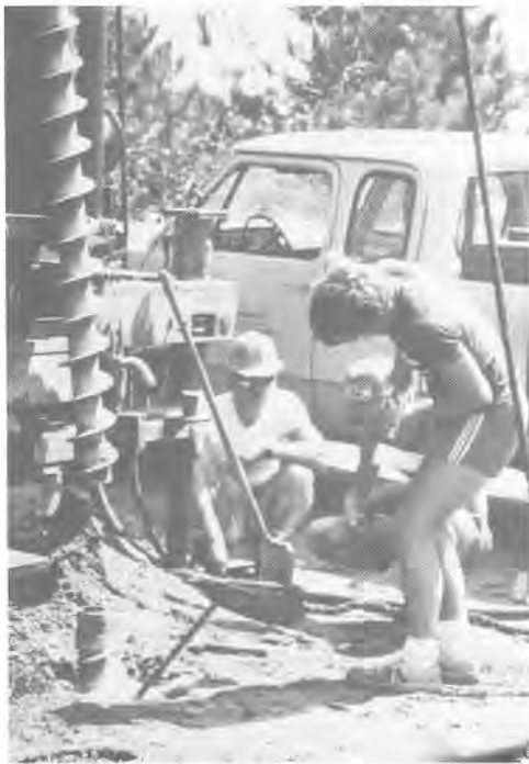
MGS geologist Craig Neil (right) and U.S. Geological Survey technicians installing a monitoring well for the Significant Sand and Gravel Aquifers project (1985).
