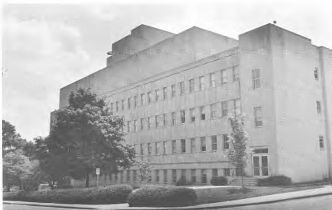
Figure 9.--Geology Building on the Indiana University campus in Bloomington; only Geological Survey wing shown.
