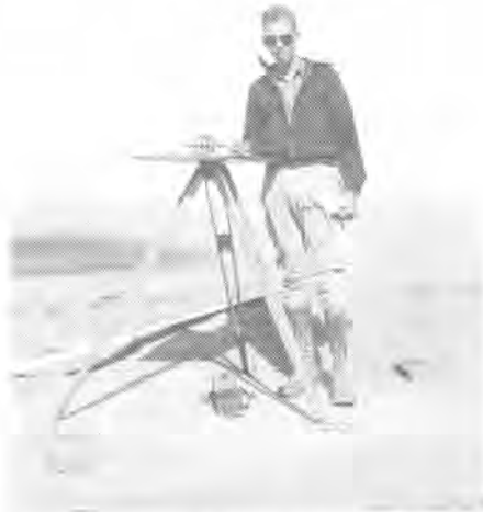
Geologist using a plane table and stadia rod for geologic mapping.
