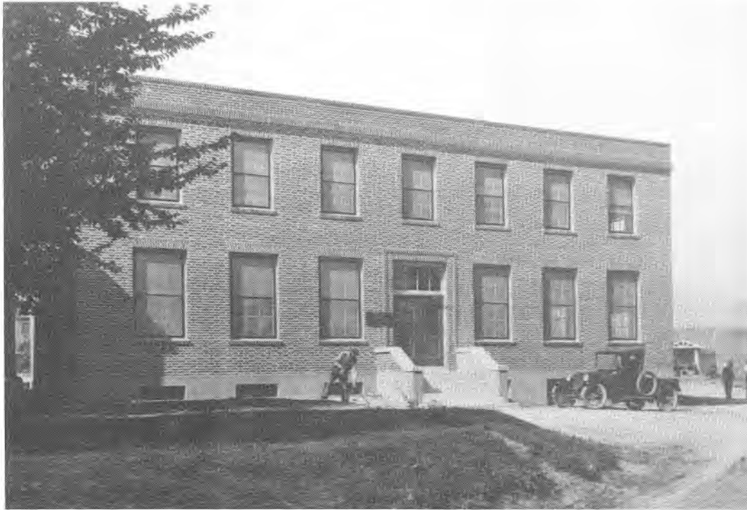
The old U.S. Bureau of Mines Experiment Station, now the Physical Plant Building, was occupied by the Nevada Bureau of Mines between 1955 and 1962. Source: UNR archives.
