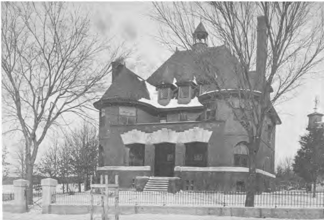
Formerly the headquarters of the Missouri Bureau of Geology and Mines from 1901 to 1904, this building is now the Chancellor's residence of the University of Missouri-Rolla.
