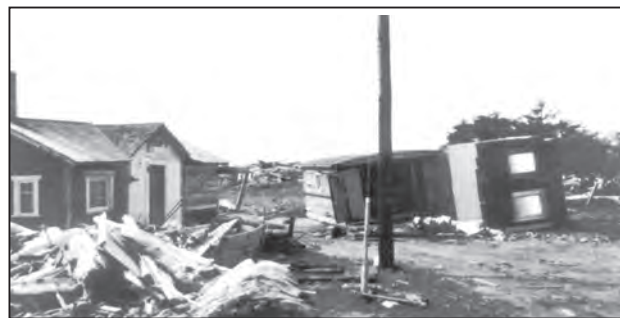
House on Washington coast destroyed by 1964 tsunami generated by Anchorage, Alaska, earthquake. From U.S. Army Corps of Engineers unpublished file report by D. W. Hogan and others (1964).
