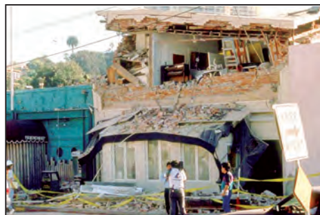
Top, Fire in San Francisco, California, after 1989 Loma Prieta (World Series) earthquake. Bottom, Damage to unreinforced masonry building from 1994 Northridge, California, earthquake. Photos courtesy Karl V. Steinbrugge Collection, University of California, Berkeley, Earthquake Engineering Research Center.
