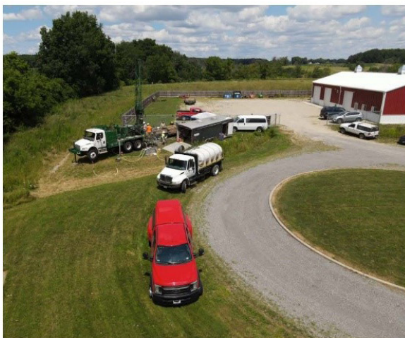
Coring, monitor well installation, purging well
